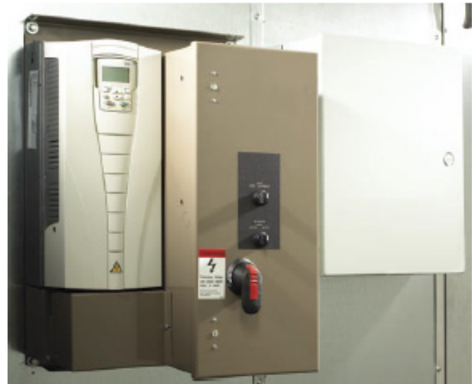
Variable-speed drives offer dramatic fan-energy savings
