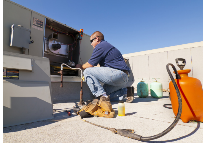
Certified technicians ready to assist jobsite installations
